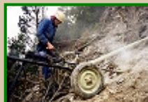
Forage au CFL
